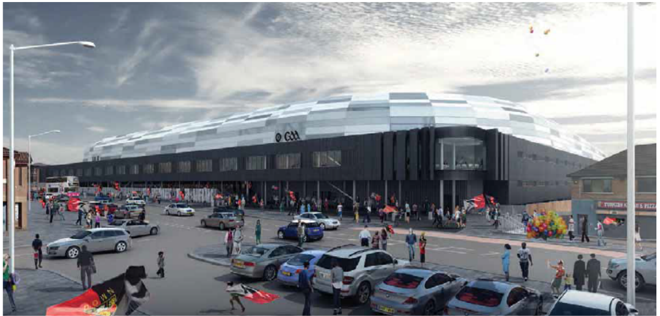
Andersonstown Road Facade looking east
